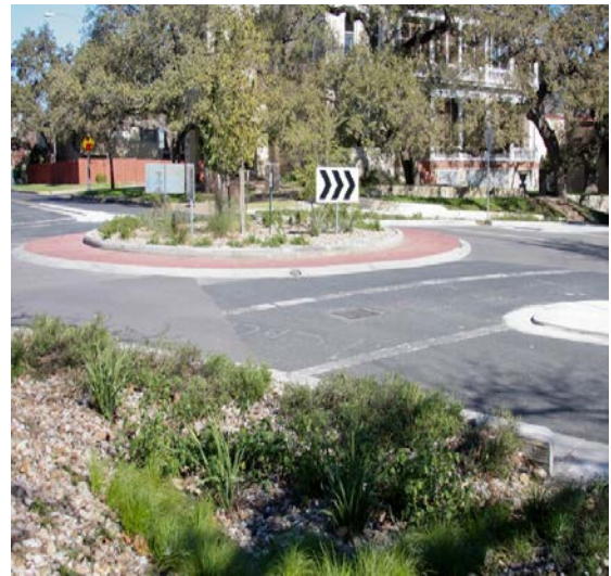
Example Roundabout with vertical enhancement. Source: NACTO
