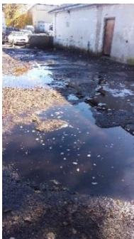
Lack of drainage on site creates swamp like ground condition
