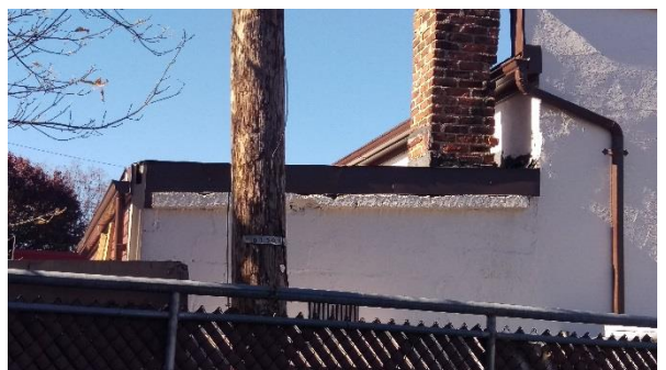
Chimney brick falling and minor flashing repairs needed
