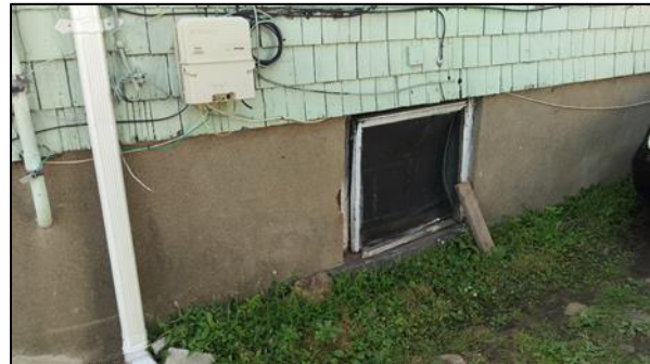
View of side – broken basement window
