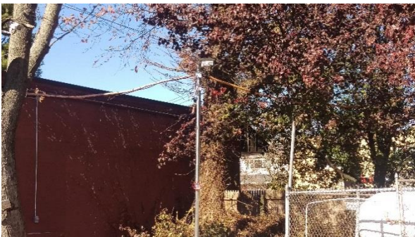
Wiring/electric from off-site to pole, then tree
