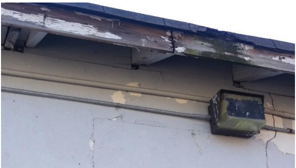
Poor soffit condition
