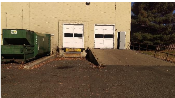
Loading area – missing railing
