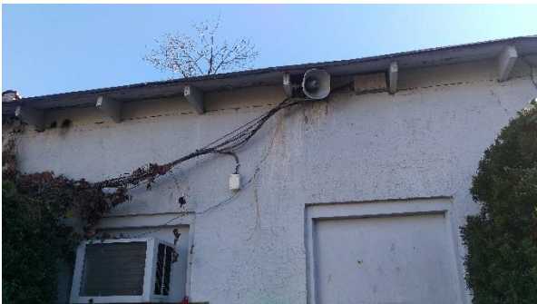
Overgrown vegetation on hanging wires & poor roof condition
