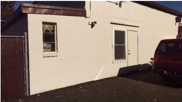
Rear of building in good condition – one broken window & 1 new window
