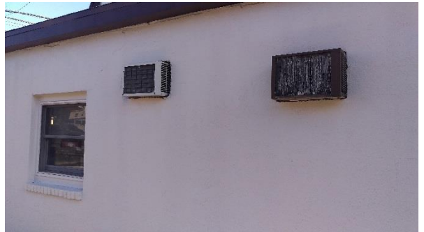
Non-tight seal around air conditioning units
