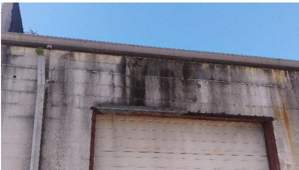
Façade damage above loading door
