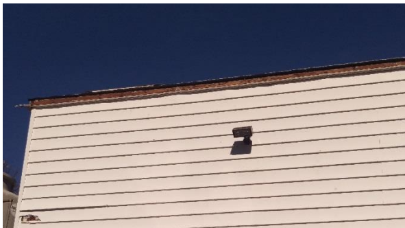
Structure above with poor soffit condition – no gutters
