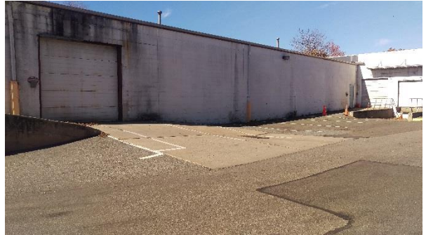
Uneven pavement in loading dock area in rear
