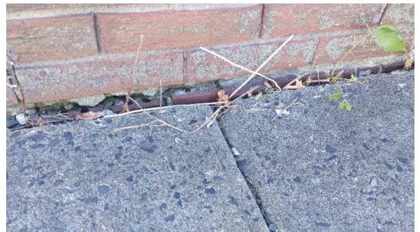
Brick separation at ground
