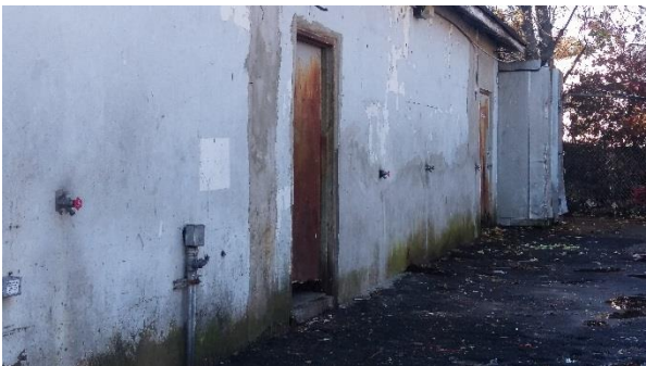
Bldg. façade & doors - mold & deterioration
