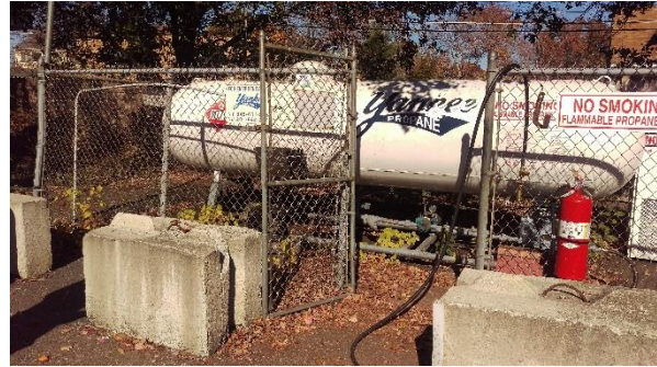
Unlatched / unsecure gate to propane tank
