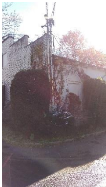
Overgrown vegetation on hanging wires & poor roof condition
