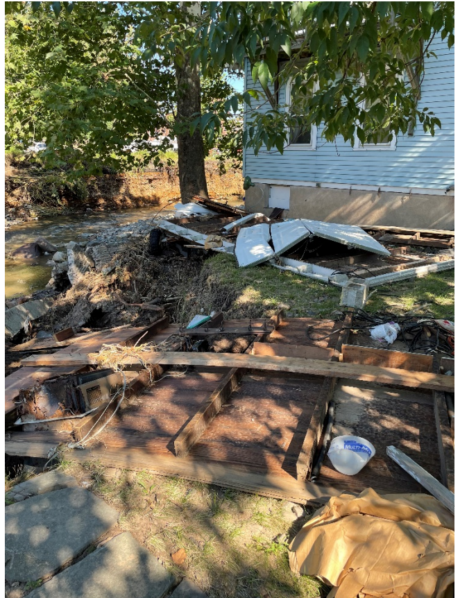
In September 2021 Hurricane Ida caused damage resulting from the flooding of Peckman Creek. Shown here is a collapsed garage and bank erosion from the incident.
